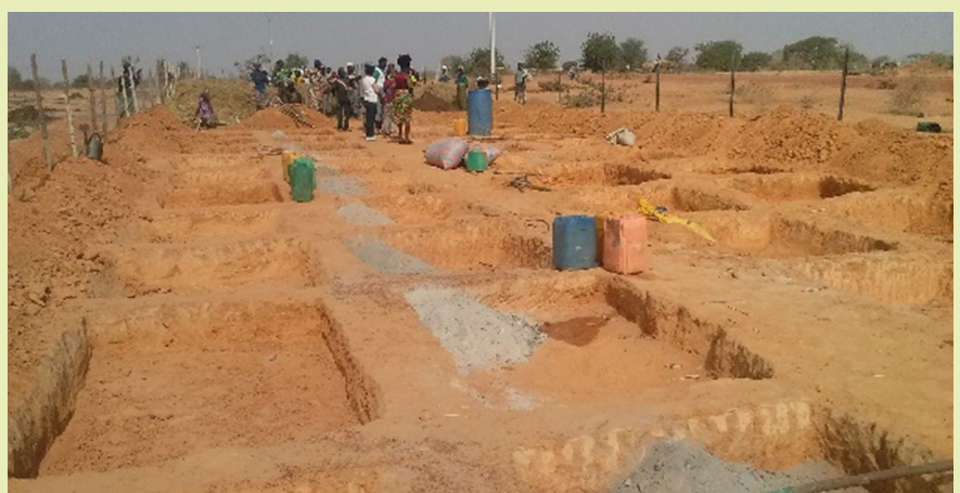
The on-site composting platform
